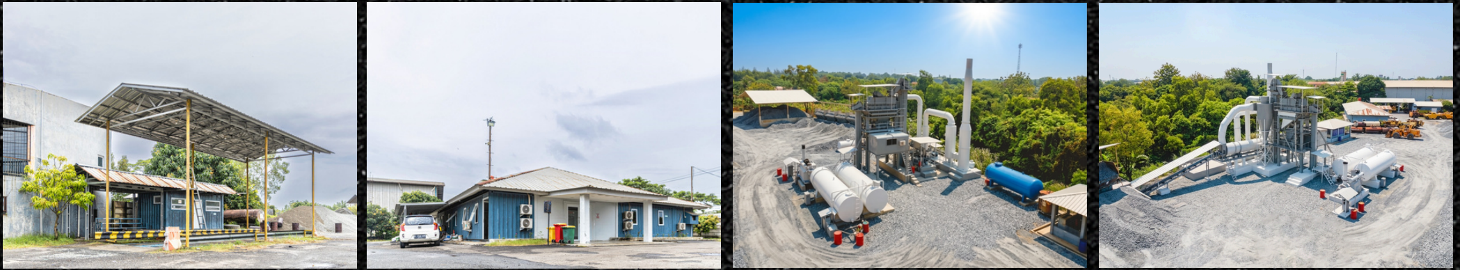
Foto Asphalt Mixing Plant
